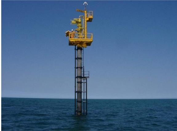
In shallow waters, typically located close to islands or the coastline, oil and gas is sometimes produced through very simple small unmanned facilities such as a “monopod” or small platform with production controlled remotely from the nearby island and with production facilities located on that island.
