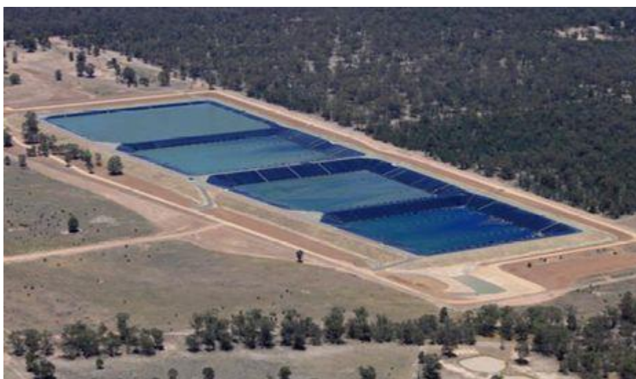
Figure 1. CSG ponds using geosynthetic liner system
