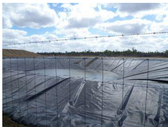
Figure 3: CSG pond under construction with fence and liner
